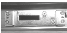
Sill Keep (double doorsets)
