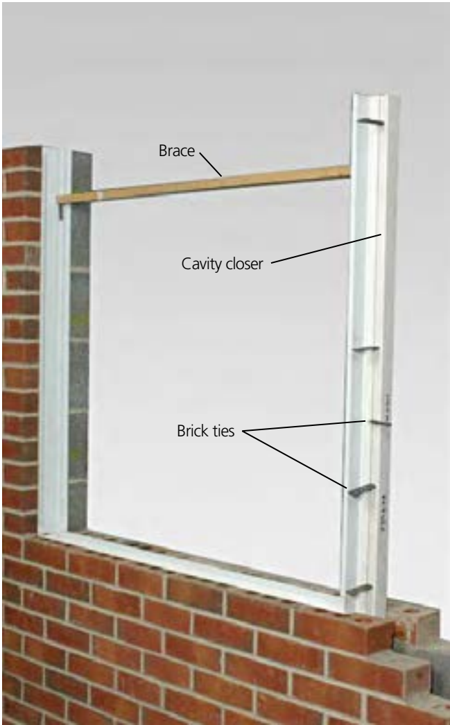
In check installation detail
