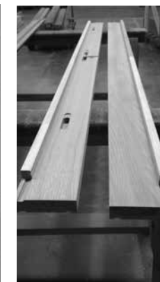
Keep Jamb and Hinge Jamb
